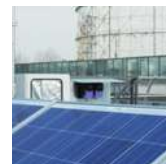
ITALY Cooling loop flow & temperature control
