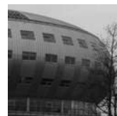
HOLLAND Hot water pumping across district network
