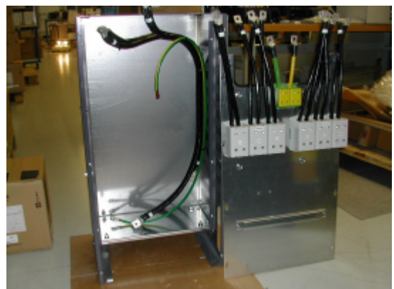
Mounting plate removal
