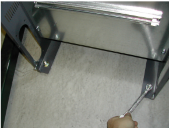
Complete unit mounting to floor
